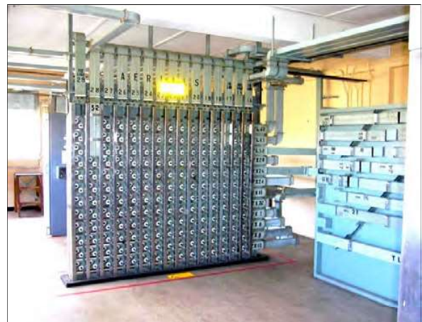
Original aerial exchange with links at right to be plugged into the aerial/transmitter matrix on the left. Photo: Keith Baker.
