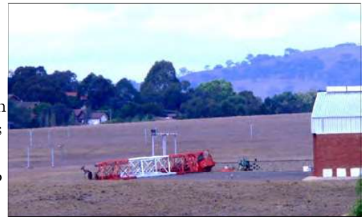
A Section of one demolished LF Tower. Photo: Keith Baker.
