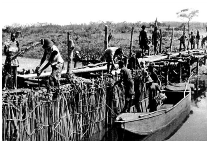
Dam building on the Dungu River to raise the river level so Corsair could escape. Source: From the internet - photographer unknown.
