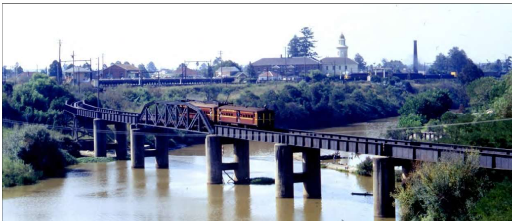
The Georges River Bridge in 1970. Liverpool station is beyond the left of the photo. The building with the tower is Liverpool Hospital. Note the plate web girder at the right is different from the rest. It came from Goulburn, the others from Rydal. Photo: Neville Hatcher ARHS 097205.
