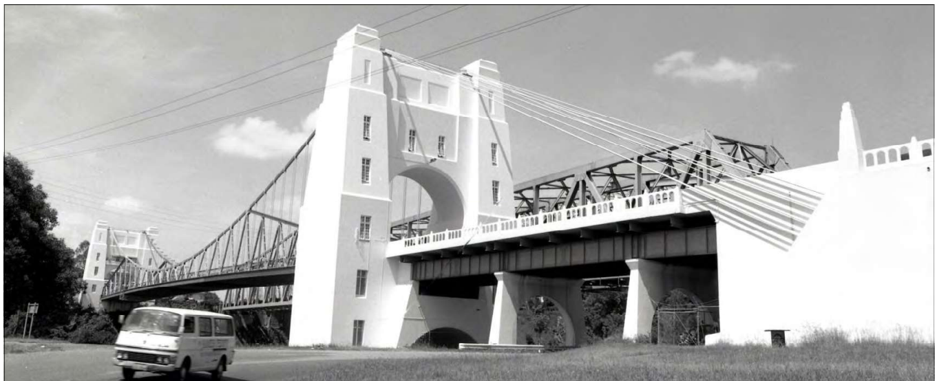
An undated, but fairly recent photograph of the Walter Taylor Bridge, viewed from the south-west. The trusses in the background belong to the adjacent railway bridge. Photo: BCC-B120-6152.
