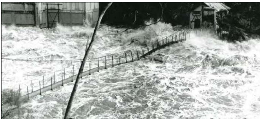
The 1929 flood. The suspension bridge was washed away. The Duck Reach Power Station building (top left) was inundated and damaged, plunging Launceston into darkness.
