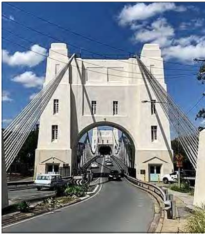
The bridge photographed in 2019, featuring a freshly painted (?) pylon. Photo: Wikipedia.
