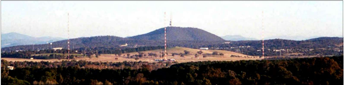
Belconnen Naval Transmitter Station, viewed from Gungahlin, before demolition of the three Low Frequency Aerial masts.
