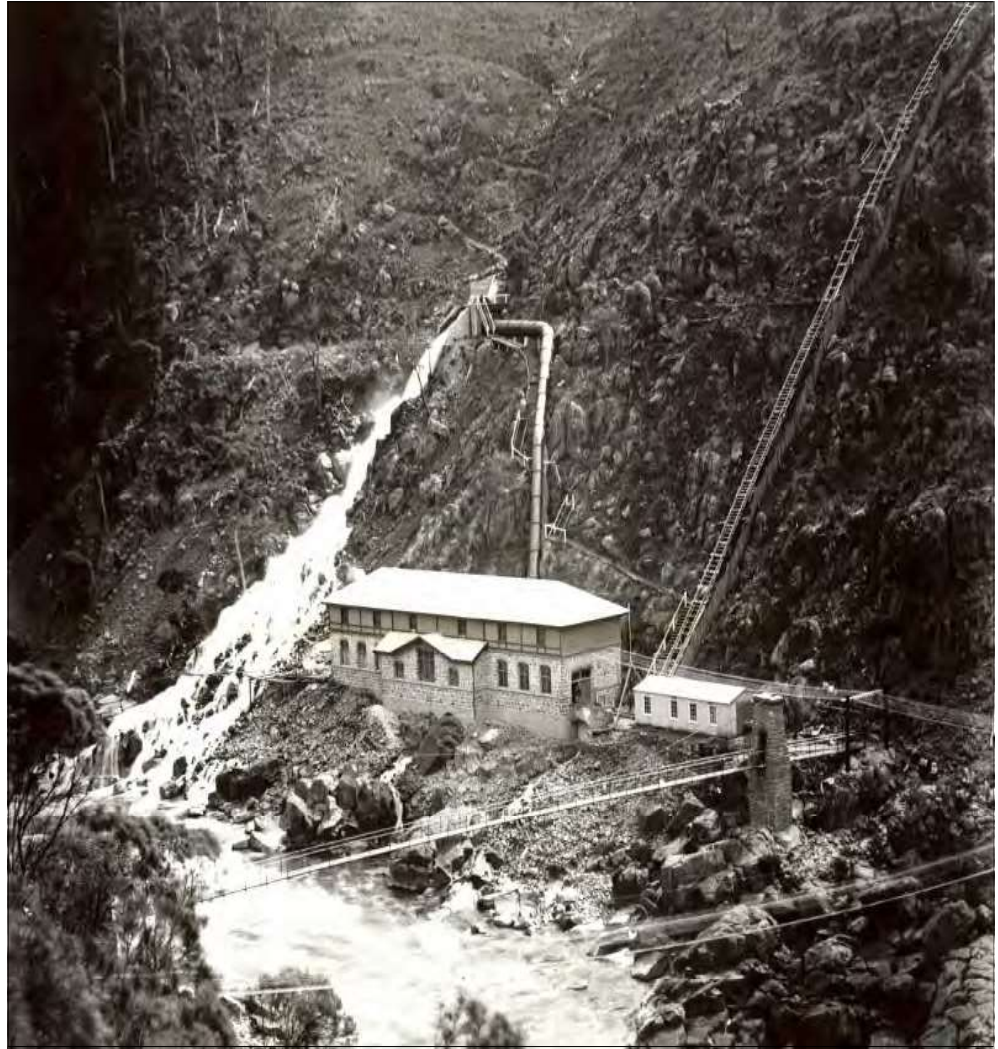
This 1905 photograph of the Duck Reach Power Station building, shows the penstock, the timber haulageway used to bring the machines down from above, and a suspension footbridge over the South Esk River. Source not provided.
