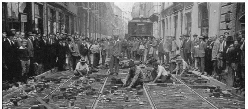
Laying wood block paving on San Pietrini, Rome, c1910.
