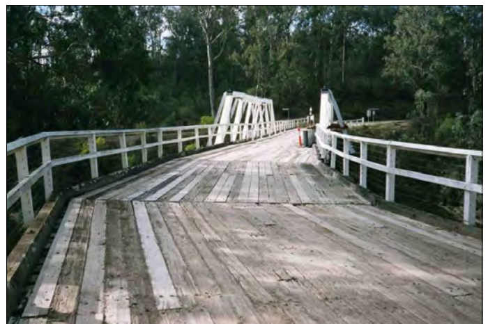
Murrindal River truss bridge decking, Buchan East, 2004.
