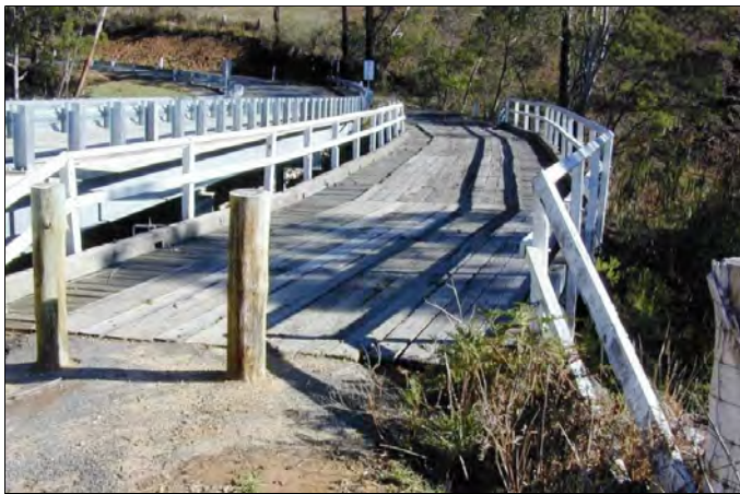
Bete Bolong Creek bridge, showing the curved decking and the new steel and concrete bridge alongside, 2003. Source: H. Martin for EGSC.
