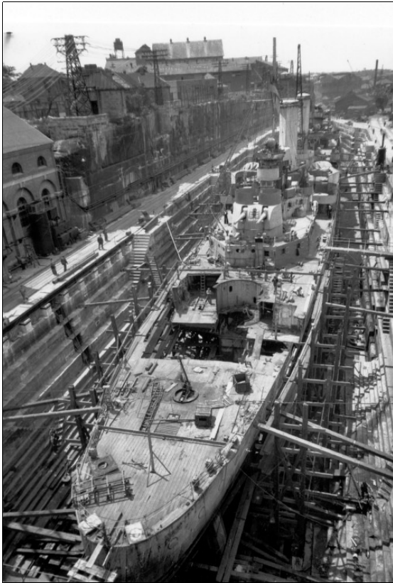
HMAS Hobart in the Sutherland Dock during her battle damage repairs in 1943. Source: J Jeremy collection.
