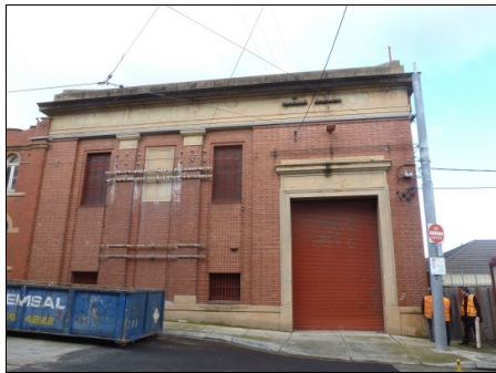
The Substation Building viewed from Coldblo Rd. Photo - Miles Pierce.
