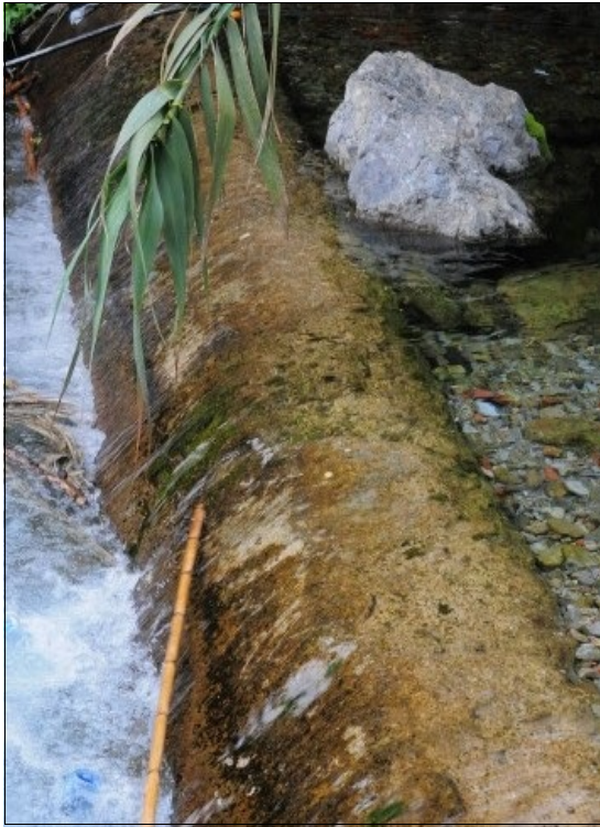
Diversion weir serving the channels to the mills.
