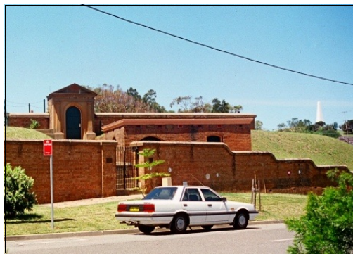
Newcastle No1 Reservoir in 1994. Photo Carl Doring.
