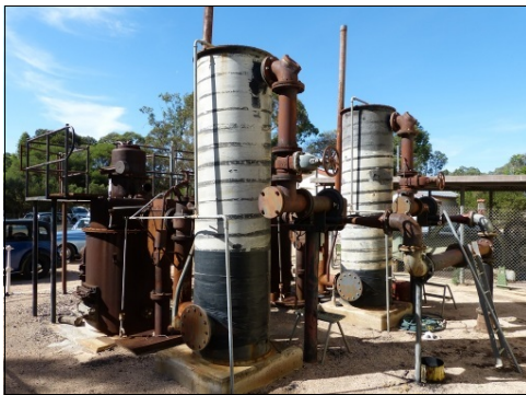
2 nd hand charcoal gas producer plant installed in 1985 after original Saunders gas producers were scrapped. Photo Keith Baker, 2014.
