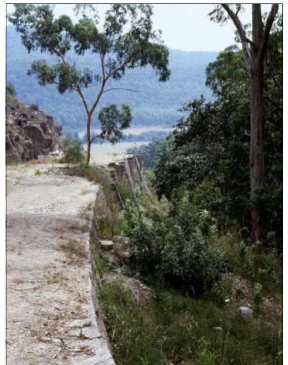
Great North Road above Wisemans Ferry in 1983. The feral tree has since been removed and the stonework repaired. Photo M. Doring.
