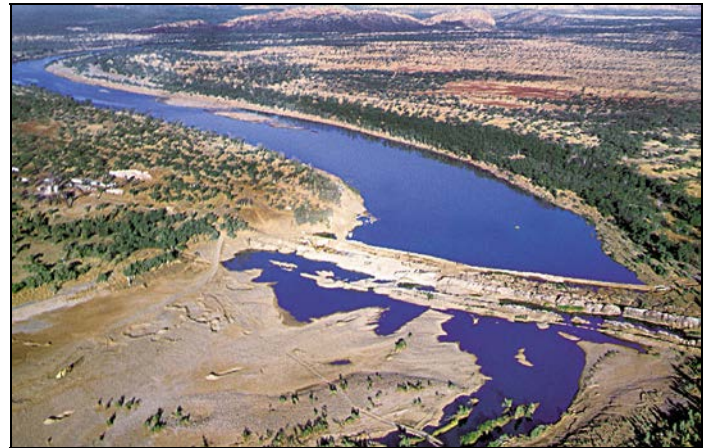
The Bandicoot Bar on the Ord River in late 1960, before dam construction started. Site offices, workshops and a concrete plant are visible on the East bank. Photo courtesy J. Lewis.
