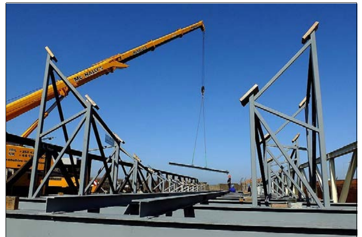
Test assembly of the Adelaide's specially designed Shipping cradle in March 2012.
