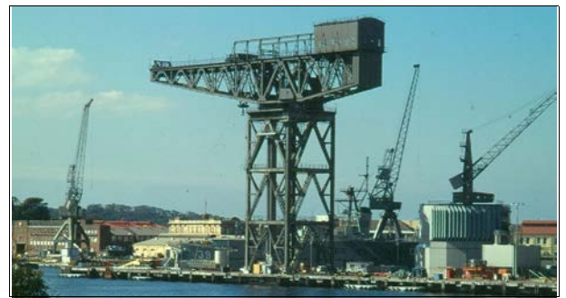
The Hammerhead (Titan) Crane at Garden Island Sydney Harbour From the National Trust (NSW)
