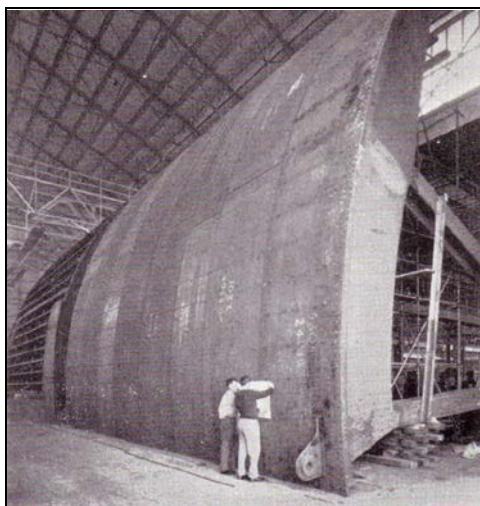
Radial gates trial assembled in Vickers Hoskins' Perth workshop. Photo courtesy Water Corporation of WA.
